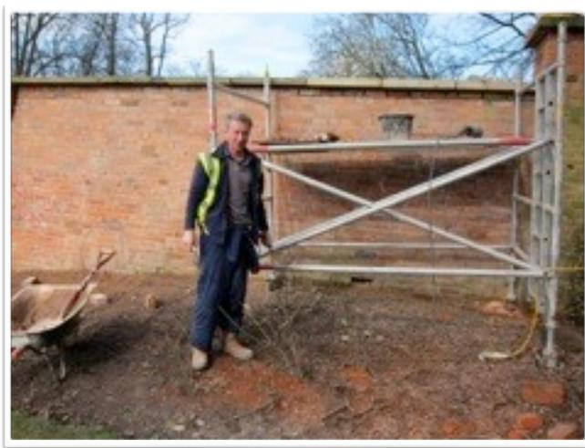
Here is Ross of E.R.M. on the final day of work on the wall. Ross told me that over eight weeks broken bricks have been replaced by matching bricks and the top six layers of brickwork have been repointed. New copings have been added so the fine old wall is now stable and secure. Good for another 150 years?
